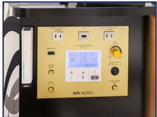
Figure 10 USB charging port beside a hotel bed [*]36 (red circle added for clarity)
